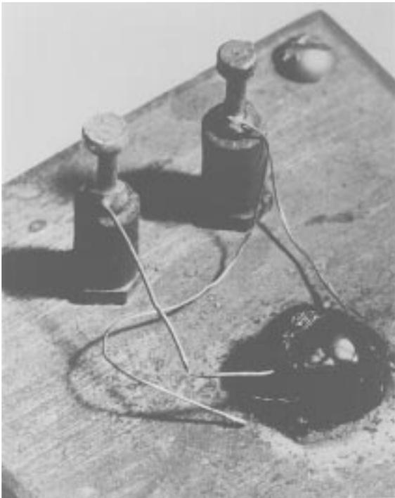
Fig. 5. Picture of the first junction transistor fabricated.
